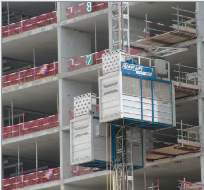
GIANT-Lift 2260FC in operation in Abu Dhabi
