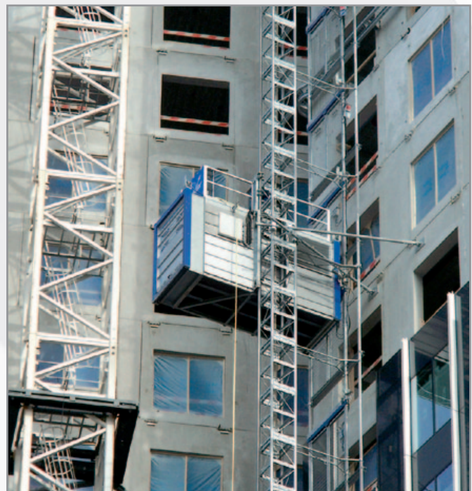
GIANT-Lift 2260FC in operation in Rotterdam
