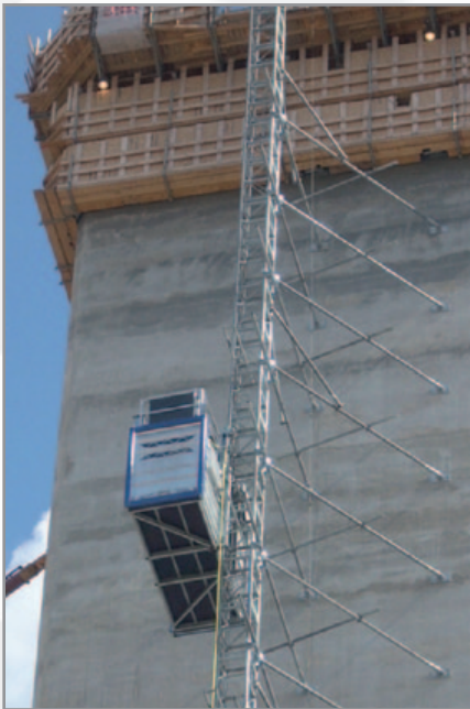
Approach of sliding formwork
